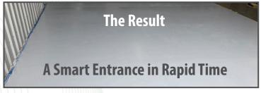
**Eracoat 2K Rapid** is a solvent free 100% solids, aliphatic coating designed as an abrasion resistant topcoat for polyurea and polyurethane systems or as stand-alone product over properly prepared substrates. It is available in 6 standard colours for a wide range of flooring and decking applications.
